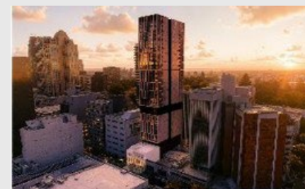
256 Queen Street Commenced a 638 bed PBSA development
